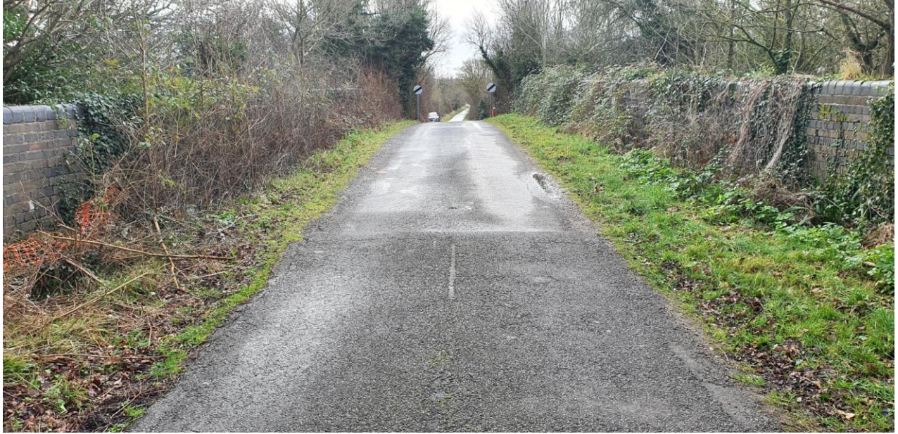
Plate A-7. View over the bridge looking south
