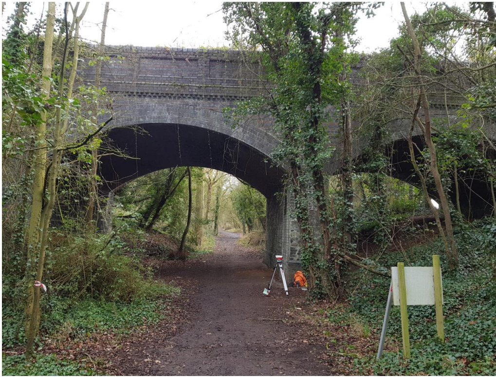
Plate A-1. View of north eastern elevation of the bridge
