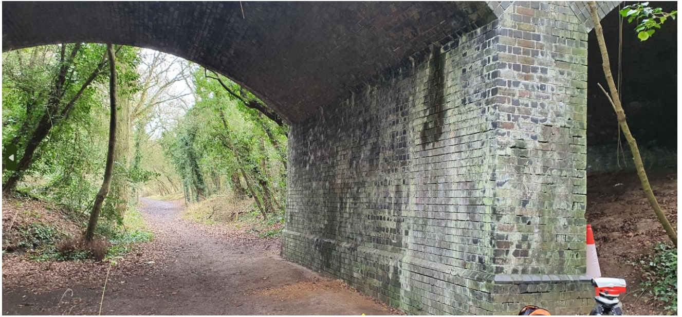
Plate A-3. View under the central arch of the bridge looking south west
