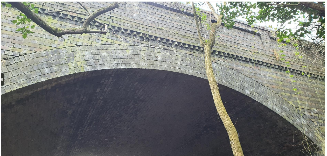
Plate A-4. View of the decorative brickwork of the central arch of the bridge
